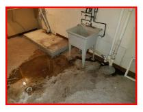
Ejector pump discharge pipe tap into cast iron waste line is bad - loose and with active leak - recommend repair by a qualified contractor.
