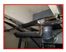
Area off water main. Copper / Galvanized piping connections are noted without the use of proper dielectric unions. Contact between copper and galvanized piping can cause corrosion in copper piping system. Recommend further review by a qualified plumbing contractor.
