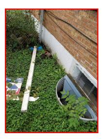
Downspouts discharge too close to building foundation. Water draining against foundation can cause serious damage to structure and water leakage into basement over time. Route downspouts away from the building as possible, ten feet is recommended. Consult a basement waterproofing contractor or a qualified landscaping professional for options on correcting downspout discharge.
