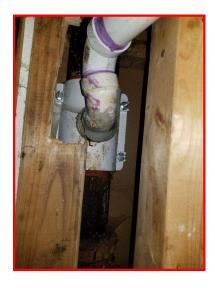
Leak noted below ejector pump discharge tap. Recommend further evaluation by a qualified contractor. Mold-like staining noted below.
