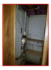
Active seepage noted at multiple spots on South wall. North wall suspect as well - but may be old stains from ejector basin area plumbing issues.
