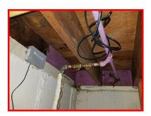
Ceiling area wet - see basement family room notes - recommend further evaluation by a qualified contractor of piping run thru area for leak. Noted reduced flow with multiple fixtures on. Recommend further evaluation by a qualified plumbing contractor for possible galvanized piping replacement.
