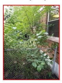
Trees are touching or overhanging the roof. Damage is possible, extra maintenance will be needed to keep roof and gutters clear of debris from tree. Recommend trimming back tree as possible.
